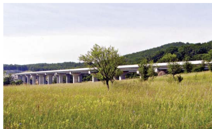
Viadukt Krpan. AC-ZG-ST Viadukt Krpan. Autobahn-ZG-ST
